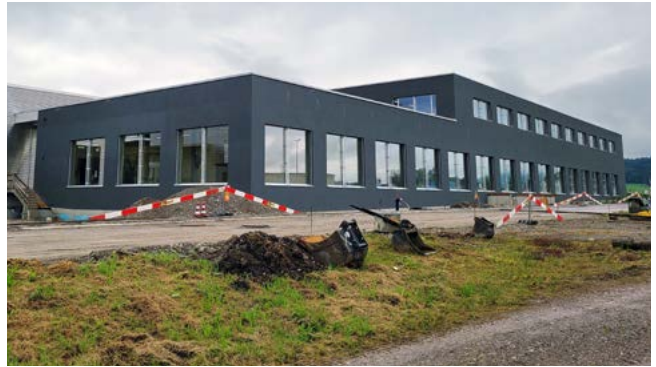
The expansion of the location of Stamm AG in Hallau (CH) was completed.
