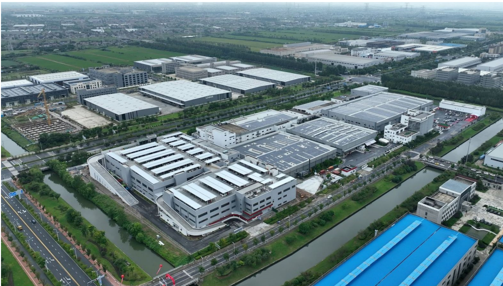
Phase two of the site expansion project in Nantong (China) was completed.
